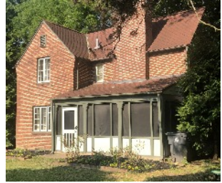
East face, caretaker's cottage.
