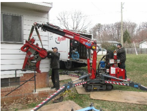
The hoisting equipment raising the 10x15" C&P at the top of the stairwell from the basement to the yard.
